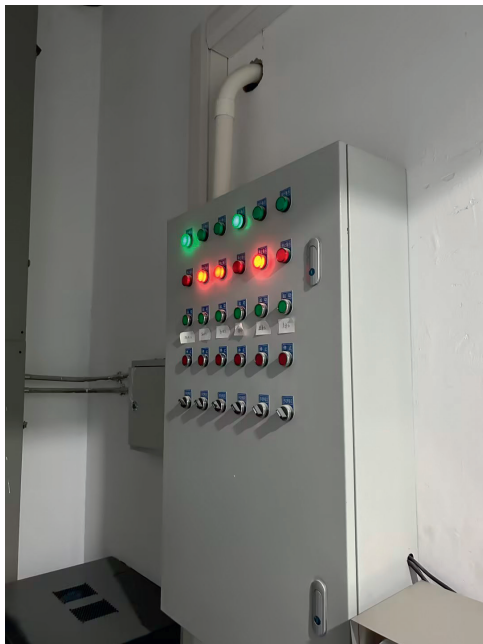
Laboratory fresh air risk control system of 3D Medicines (Beijing) 思路迪(北京)實驗室新風控制系統
