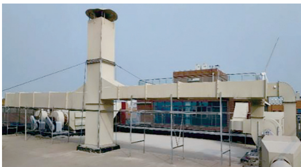
3D Medicines Beijing Laboratory exhaust gas treatment device 思路迪北京實驗室廢氣處理裝置
